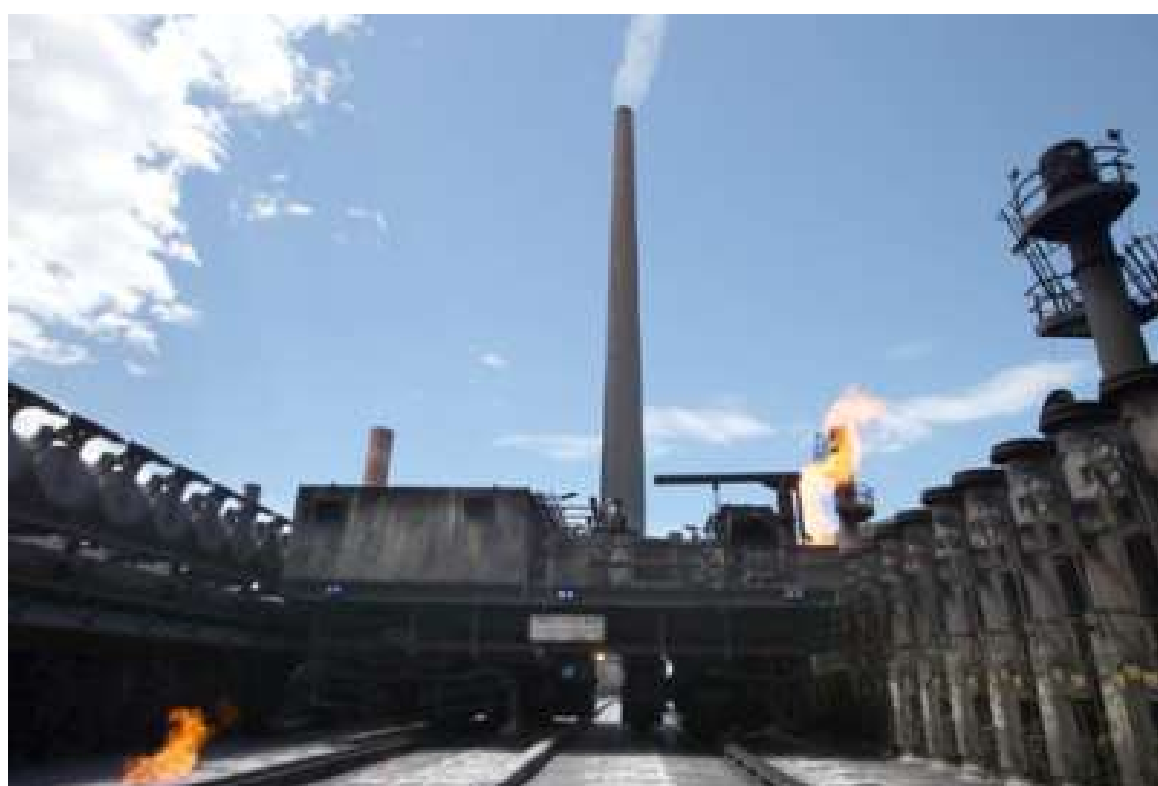
Reforma de coqueiras Coke plant repair
