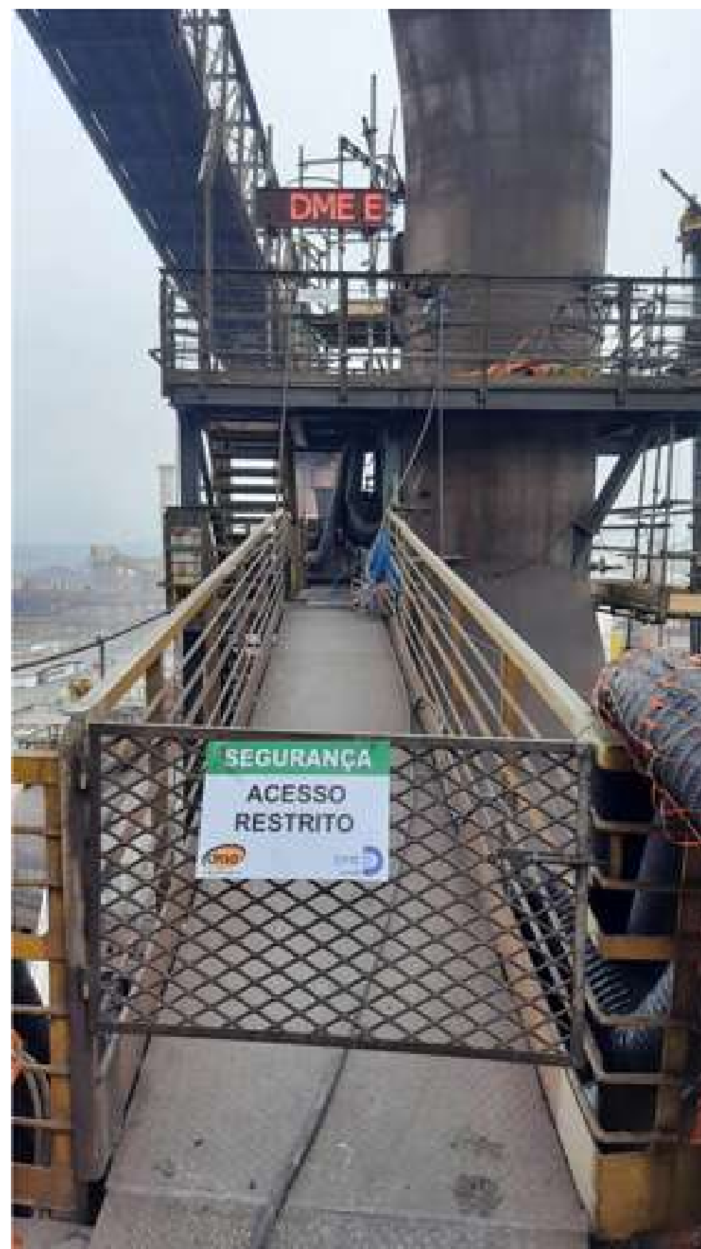
Reparo mecânico e refratário do downcomer Downcomer mechanical and refractory repair
