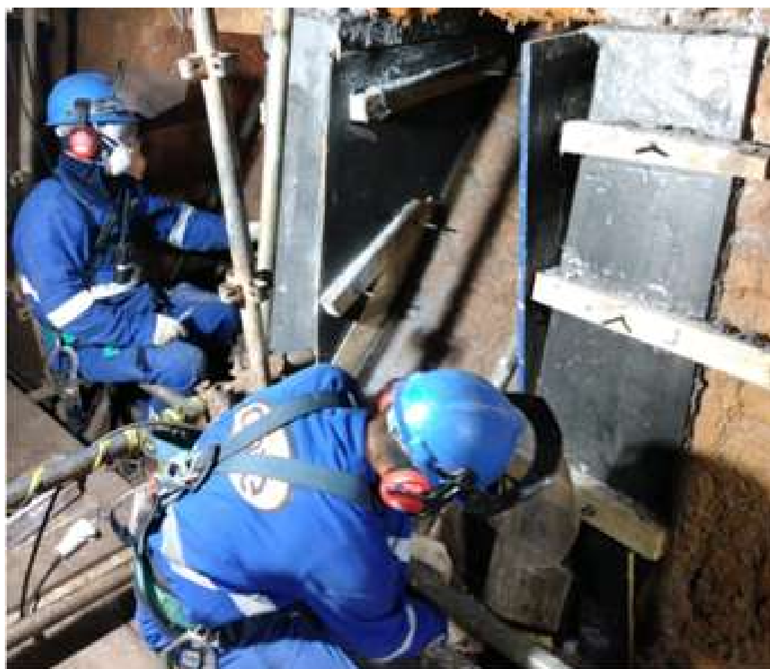
Reparo de caldeiras Aluminum Boiler repair
