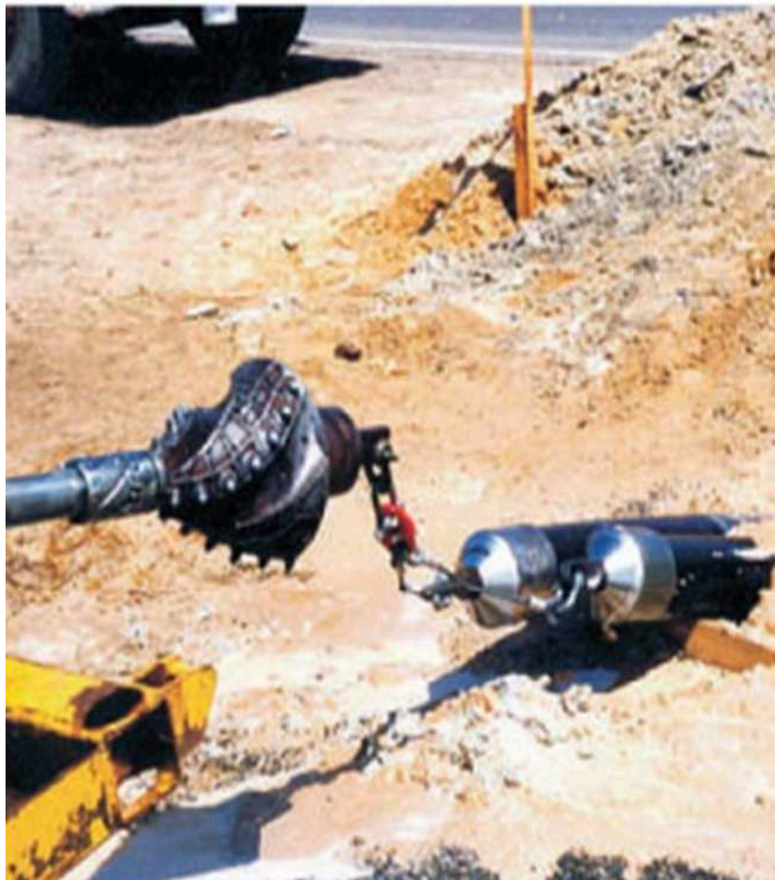
Twin 42" Dia steel casing for 600m DI restrained water line - ADWEA
