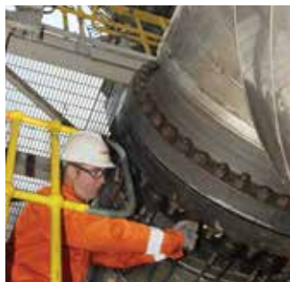
Controlled Bolting Services
