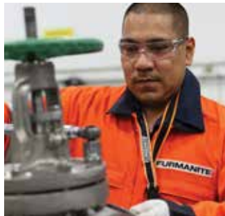
On-line Safety & Relief Valve Testing Services
