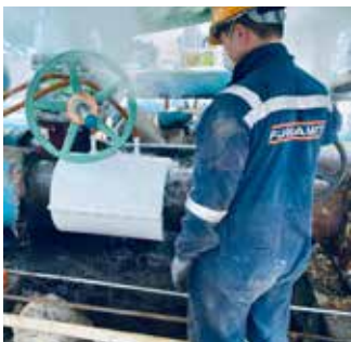
Pipe Freezing Services
