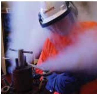
On-line Leak Sealing & Repair Services
