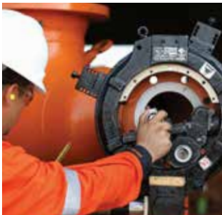
Onsite Machining Solutions
