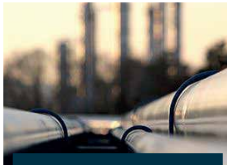
PLANT & PIPELINE MAINTENANCE
